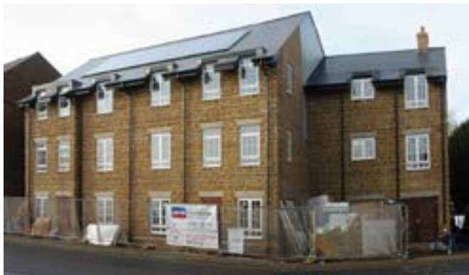
Palmer Court extension almost completed
