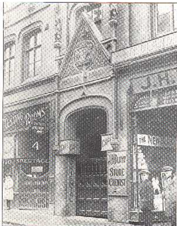
Entrance to Masonic Hall Abington Street Northampton Opened 1875
